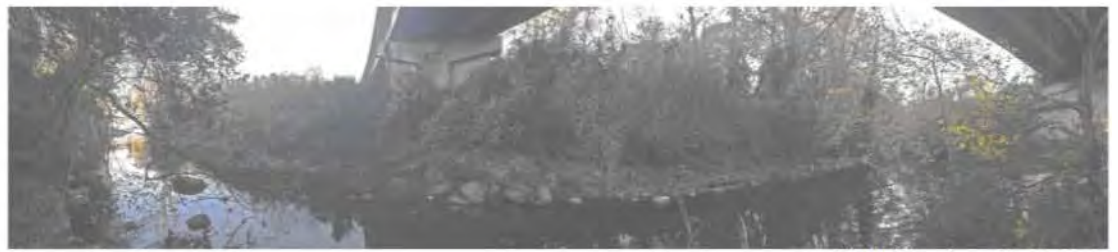
Marta Bridges Across Proctor Creek
