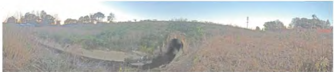
Proctor Creek Through Culvert under North Avenue
