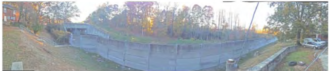
Continuous Fence Along the Rail
